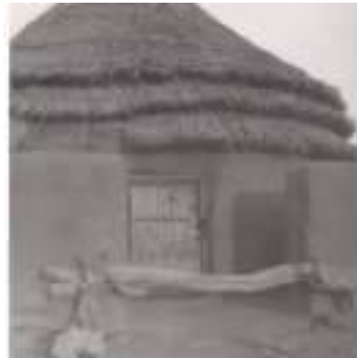
Fig 11. 3 layered thatched roof
