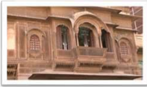
Fig.28. Typical haveli facades Source : https://www.archinomy.com/
